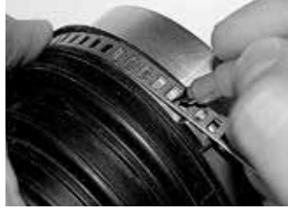
Step 2 Determine the clamp length.
