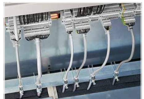
Cable entry in the base of the control cabinet Separate strain relief, movable IP54 bottom plates sealed with sponge rubber (e.g., by Rittal)
