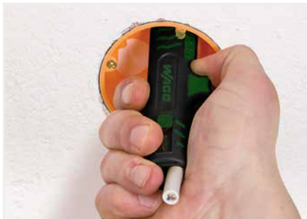
Stripping a cable sheath.
