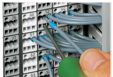
Terminating ferruled conductors via operating tool.
