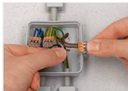
Termination: Insert the stripped solid conductor until it hits backstop.
