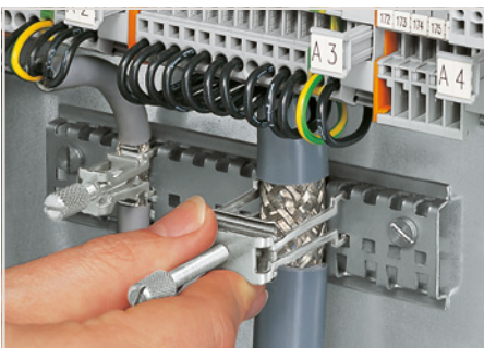
Securing an additional shield clamping saddle.
