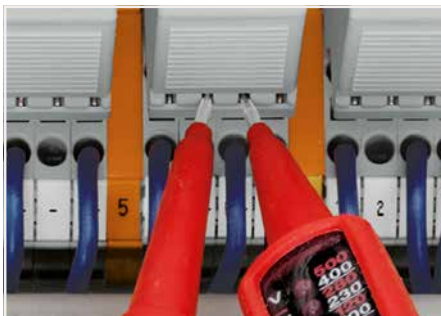
Function testing via touch-proof test slots.
